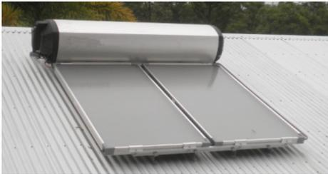
Cyclone Marcia and the failure of notifiable work audits have placed the mounting of solar water heaters in the spotlight, specifically assembly of mounting frame bracket to a solar hot water storage tank and/or collector/s to building structures.
