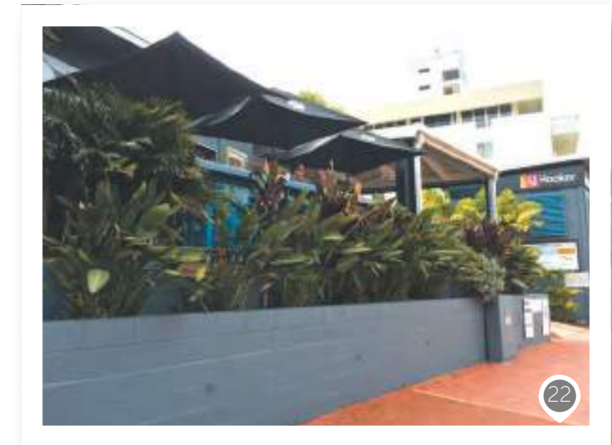
Photo 22 Normanby (Flour) [n,o,t,w,y] Comments: Effective use of landscaping to address a substantial grade difference, providing pedestrian interest and screening for outdoor dining.
