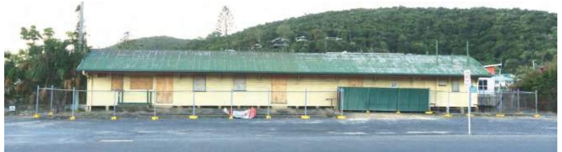
Railyard building site
