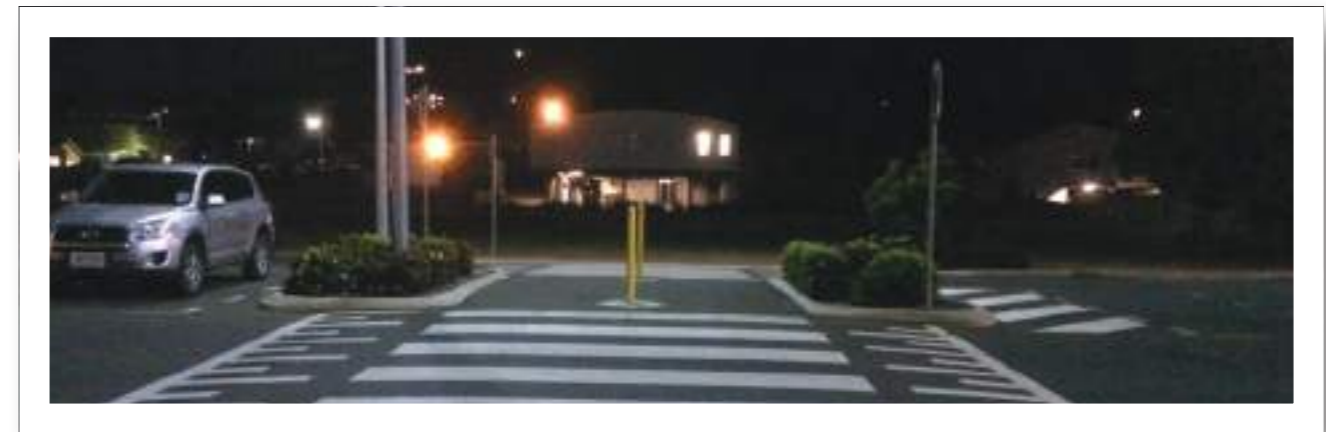
Crossing on James. Well lit, but lighting levels either side are problematic.
