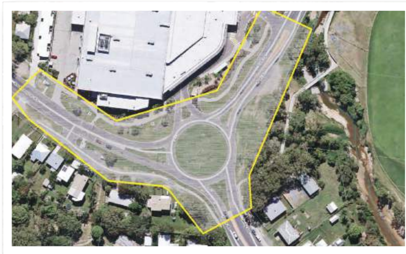
Figure 21. Roundabout at intersection of Park Street, Tanby Road and Rockhampton Road
