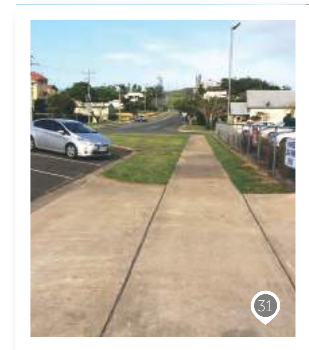
Photos 30,31 Existing footpaths, south side of John Street, looking west and east from front of Council facilities.
