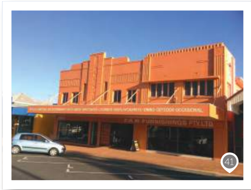
Photo 41 James Street [n,s,u] Comments: One of Yeppoon's signature art deco structures. Restoration of original colours would be preferable although the building works well in its current format because the colour is engaging, the building's key features have been retained, and the commercial signage is subtle. Accent lighting and curb-side landscaping would provide additional value-add.
