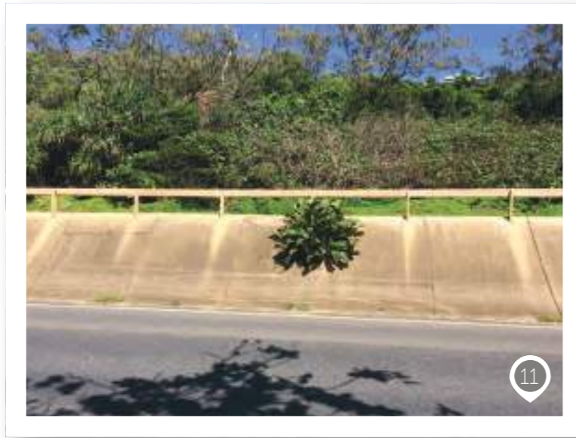
Photo 11 Sloped concrete centre median illustrating planter hole
