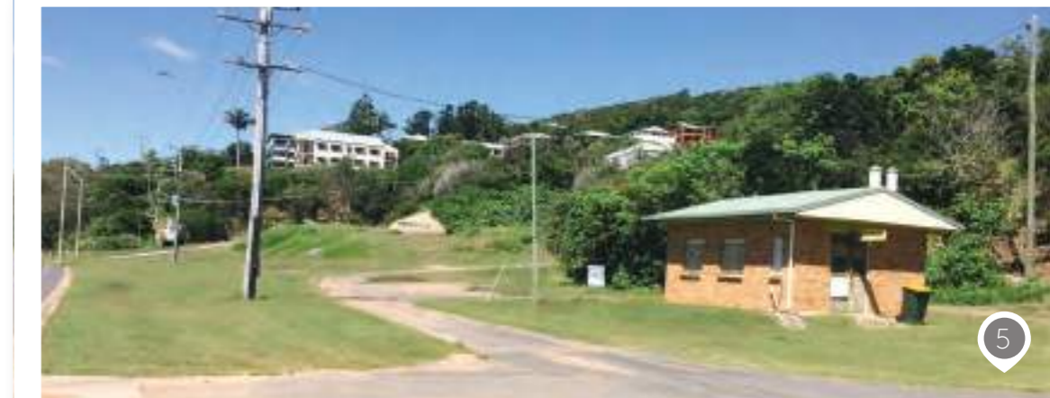
Photo 5 Council-controlled property north of the Bluff on Farnborough Road (south view)
