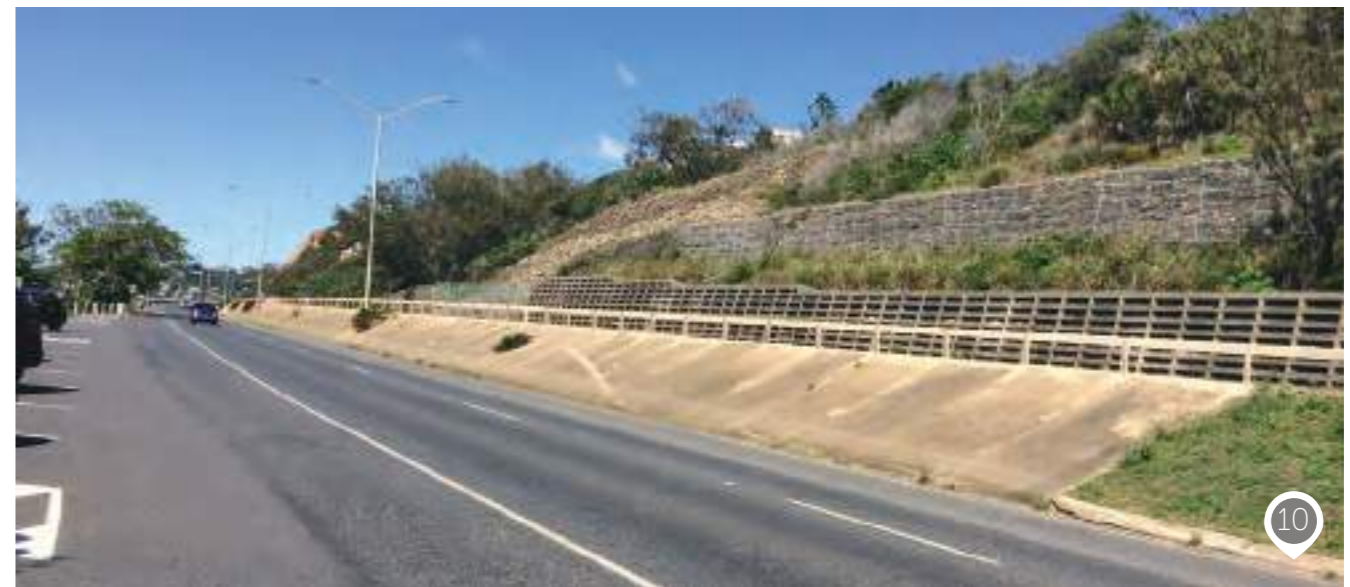
Photo 10 Sloped concrete centre median of Farnborough Road approaching Yeppoon
