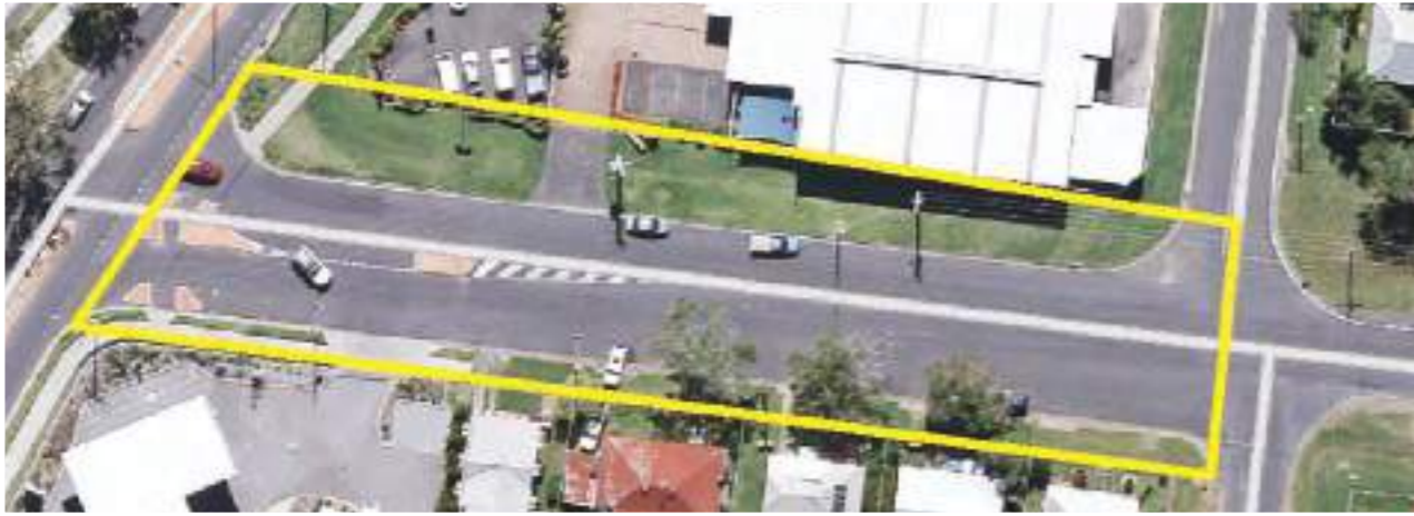
Figure 13. John Street, Park to Morris
