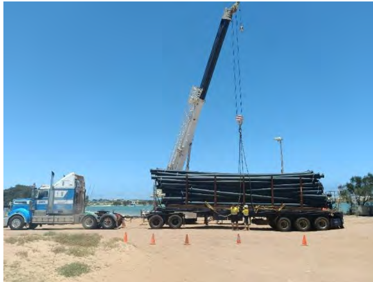
Figure 6-17 Unloading of pipe racks from semi-trailer
