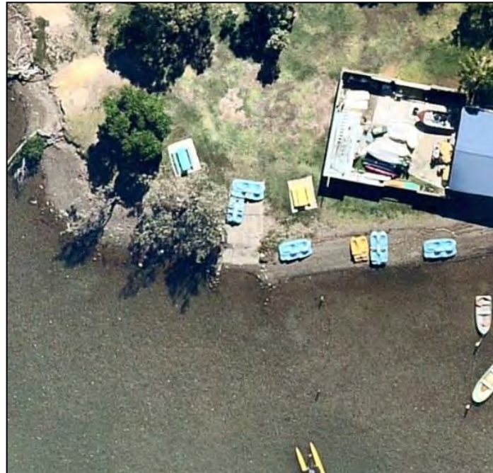
Figure 3-4 Boat Shed Ramp
