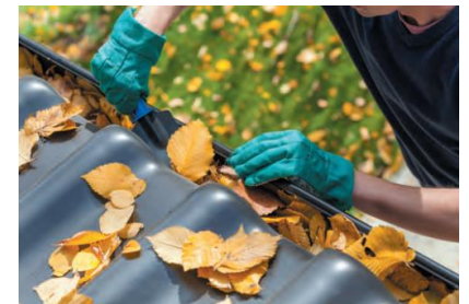
Regularly clean Debris from your gutters.
