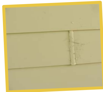
Hardi plank wall sheeting
