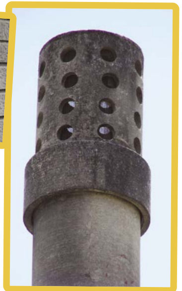
Vent pipe cap and socket fitted over a vent pipe
