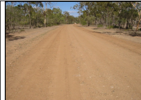
Good Gravel Pavement
